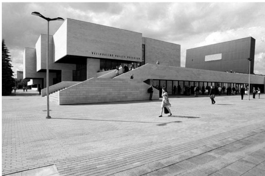
Structure after restoration Photo by Vaidotas Aukštaitis
